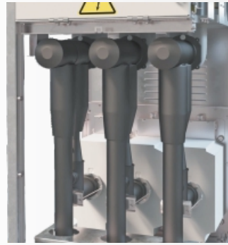
Phase current sensors for T-connectors
