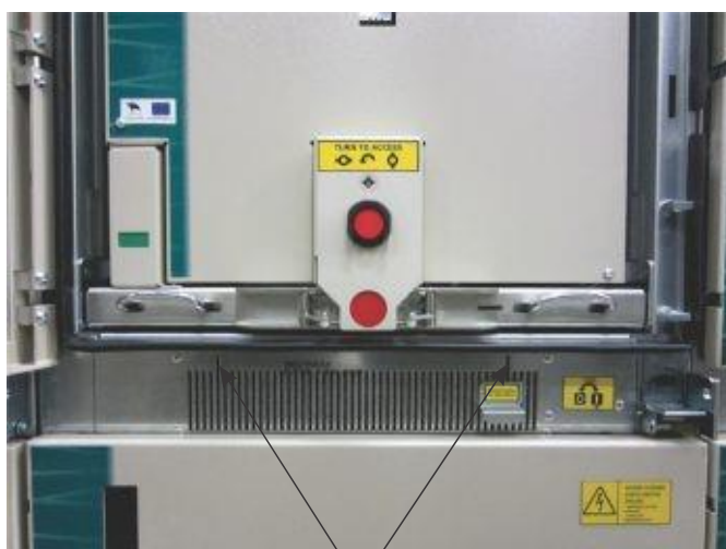
Openings for trolley guides
