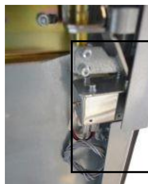
Earthing switch electromagnetic interlock
