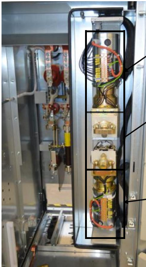
LBSF panel with motor operating devices inside
