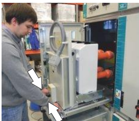
Slide 2 handles simultaneously to the middle
