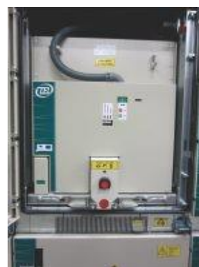
DOU is in the test position
