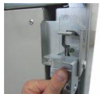
Socket for operation with earthing switch
